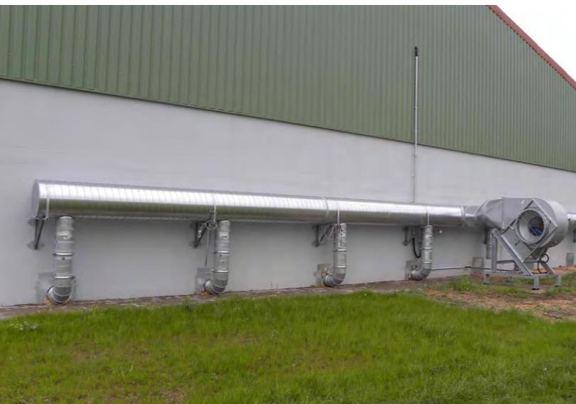
Main ventilation duct for TBR with controllable valves
