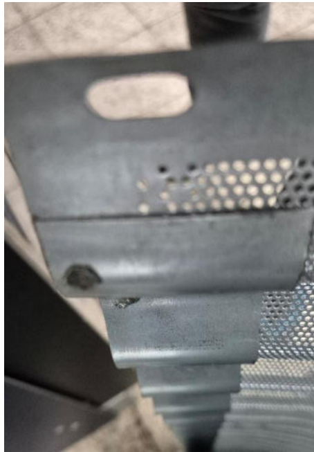
Figure 13: Stiffener on the outer tube made of perforated sheet metal must be on the inside.
