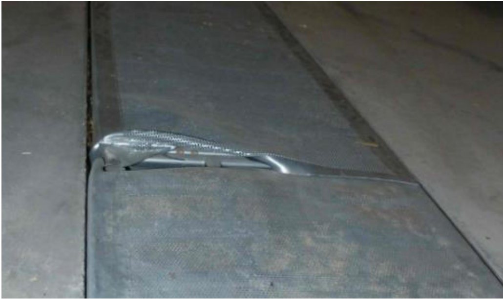
figure 6: damaged covers
