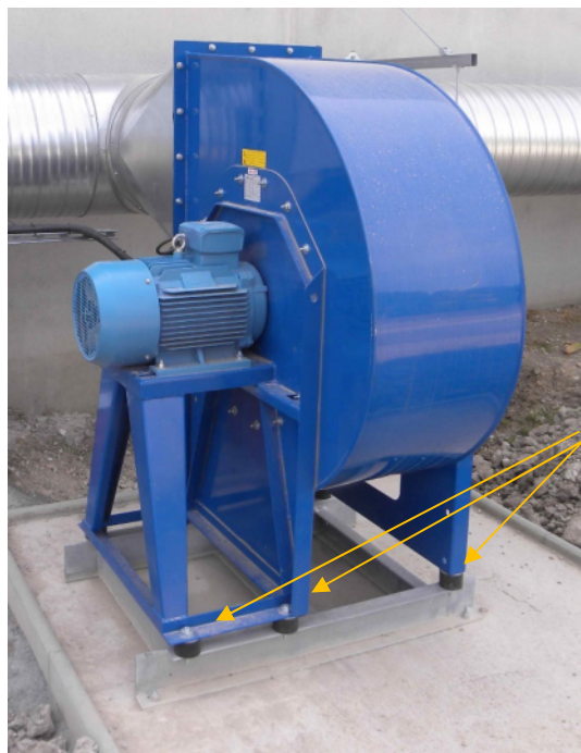
Abbildung 4: Use rubber buffers underneath the fan.
