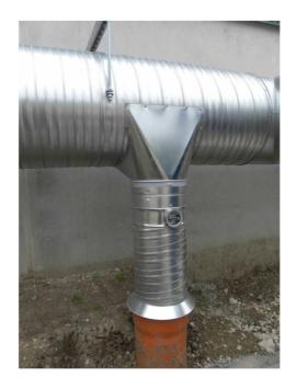
The control valve can be completely closed if necessary.
